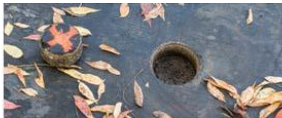
Figure 8: Remove the core from the hole
