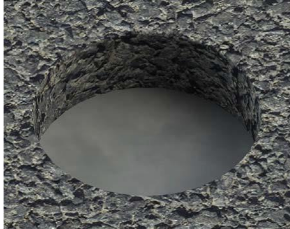
Figure 9: Bottom layer of epoxy
