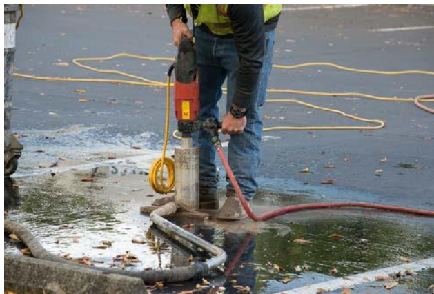
Figure 7: Drill the hole for the PlacePod
