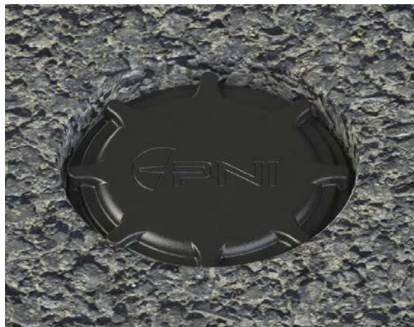
Figure 10: Sit the PlacePod in the hole (ensure top of sensor is 0.25 inches from surface)
